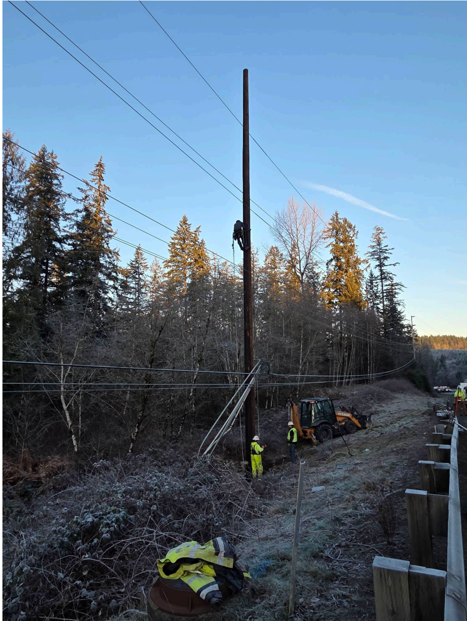
Line crew replacing transmission pole along Spirit Lake Hwy destroyed by car 01/23.
