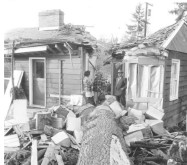
Cowlitz PUD assesses damage caused by the 1962 Columbus Day Storm
