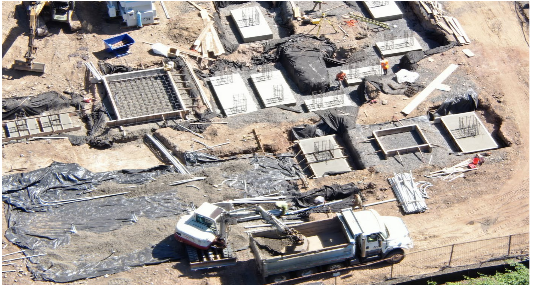
Excavation and New Foundations
