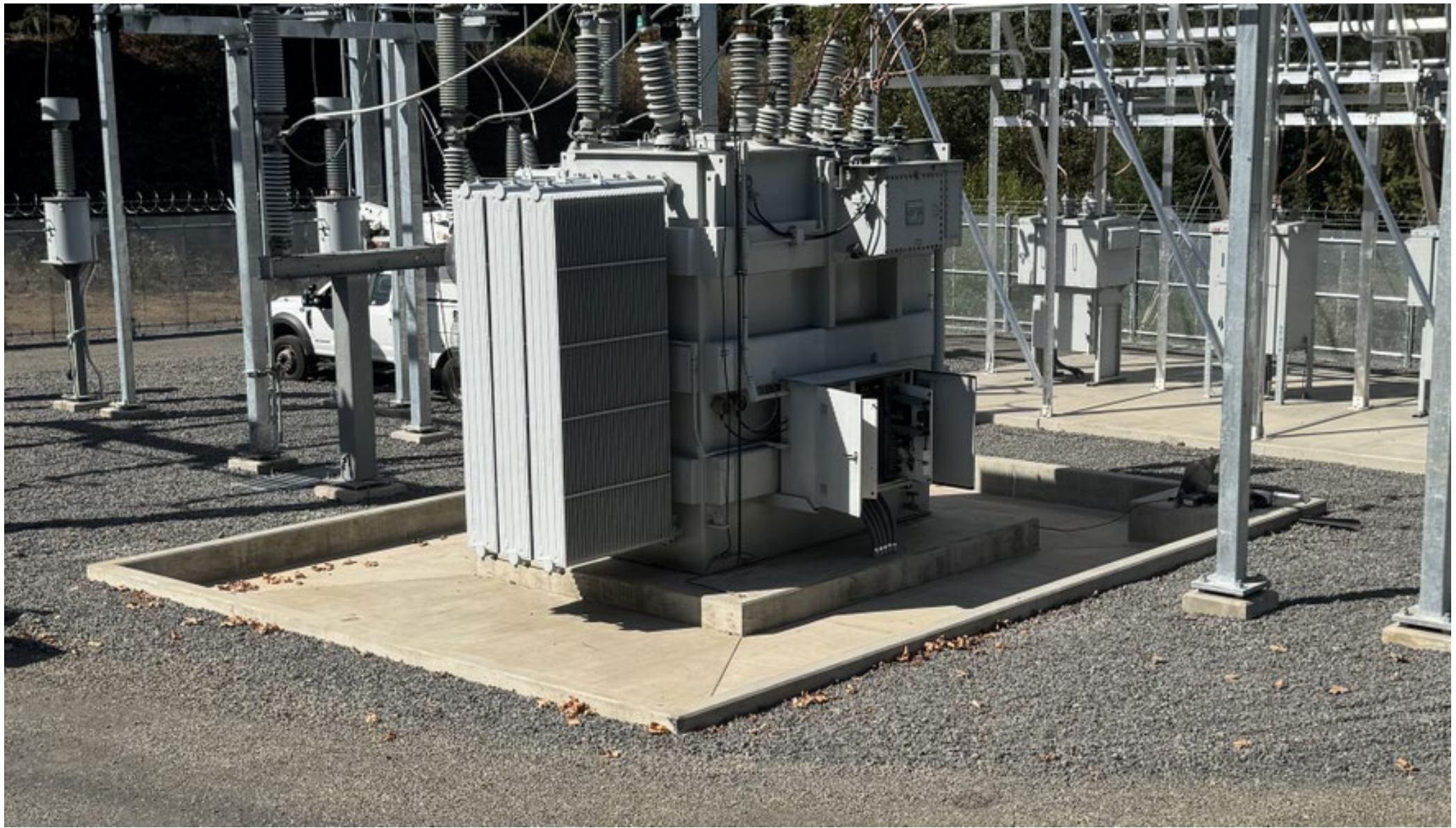
New Oil Containment and Transformer Pad
